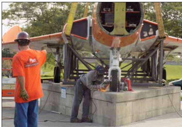
Thomarios cut a metal mount, freeing the Skylancer from its place on the platform on September 11, 2017. The crane's straps, placed through the channel on the custom-made frame, supported the plane.
