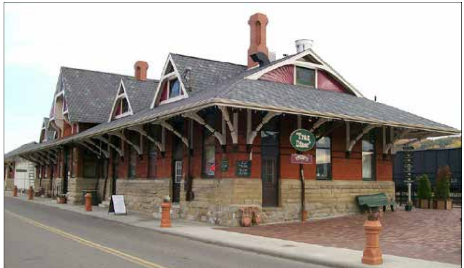
The Dennison Railroad Depot Museum and Uhrichsville Clay Museum. Photo courtesy the Dennison Railroad Depot Museum.
